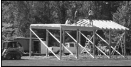
Construction of the new pavilion in the West park in 2010.
